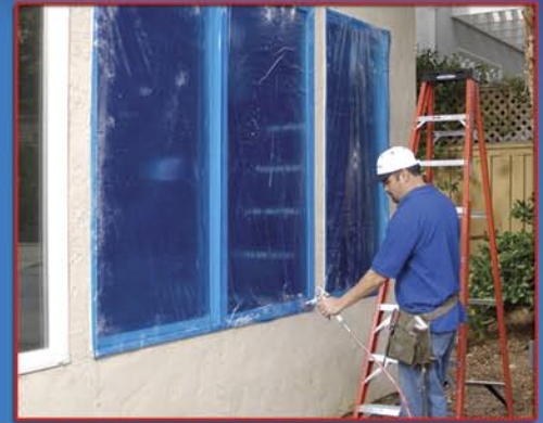
Glass being protected during stucco painting
